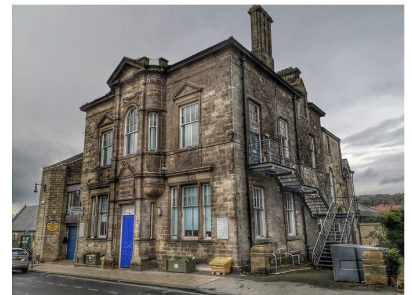
02 Former Mechanics Institute
